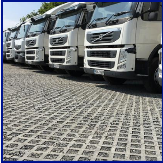
Figure 29: Truck Grid (Source: GrassMats Ltd)
