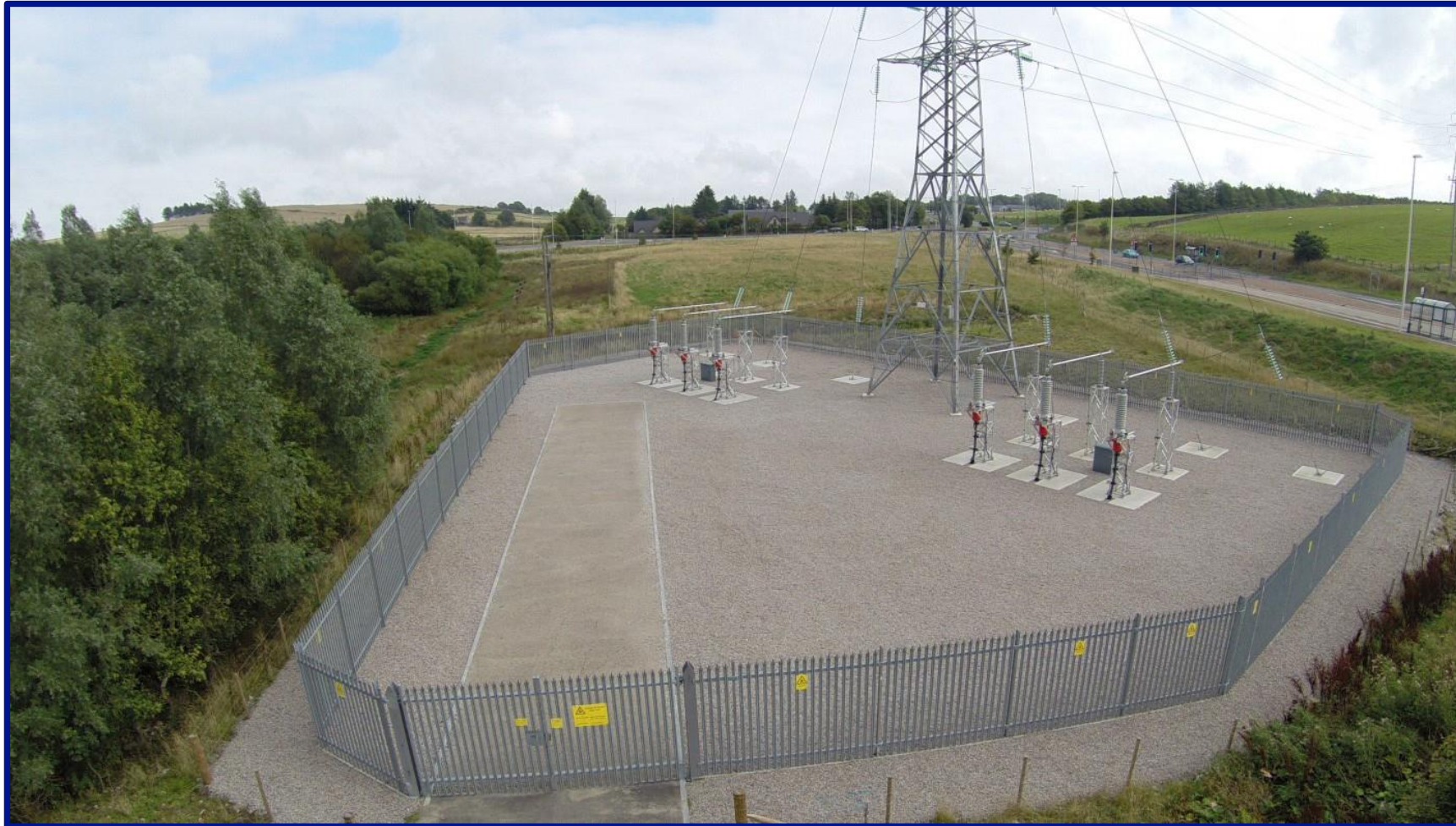
Figure 5: Existing CSE with Anchor Blocks (Source: Corrie Construction)
