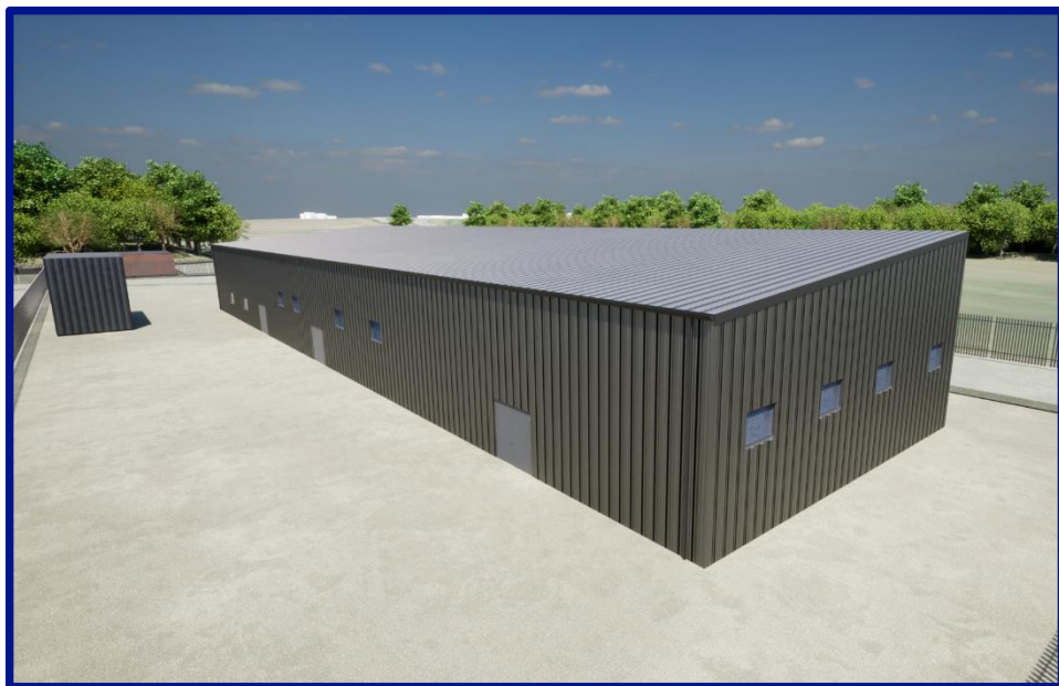
Figure 28: Overton Control Building Finish - Grey Cladding
