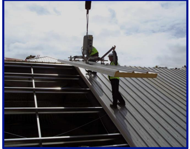
Figure 22: Grey Roof Cladding (Source: Cladco)
