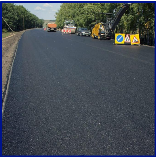
Figure 31: Impermeable Tarmac Road (Source: Swift surfacing)
