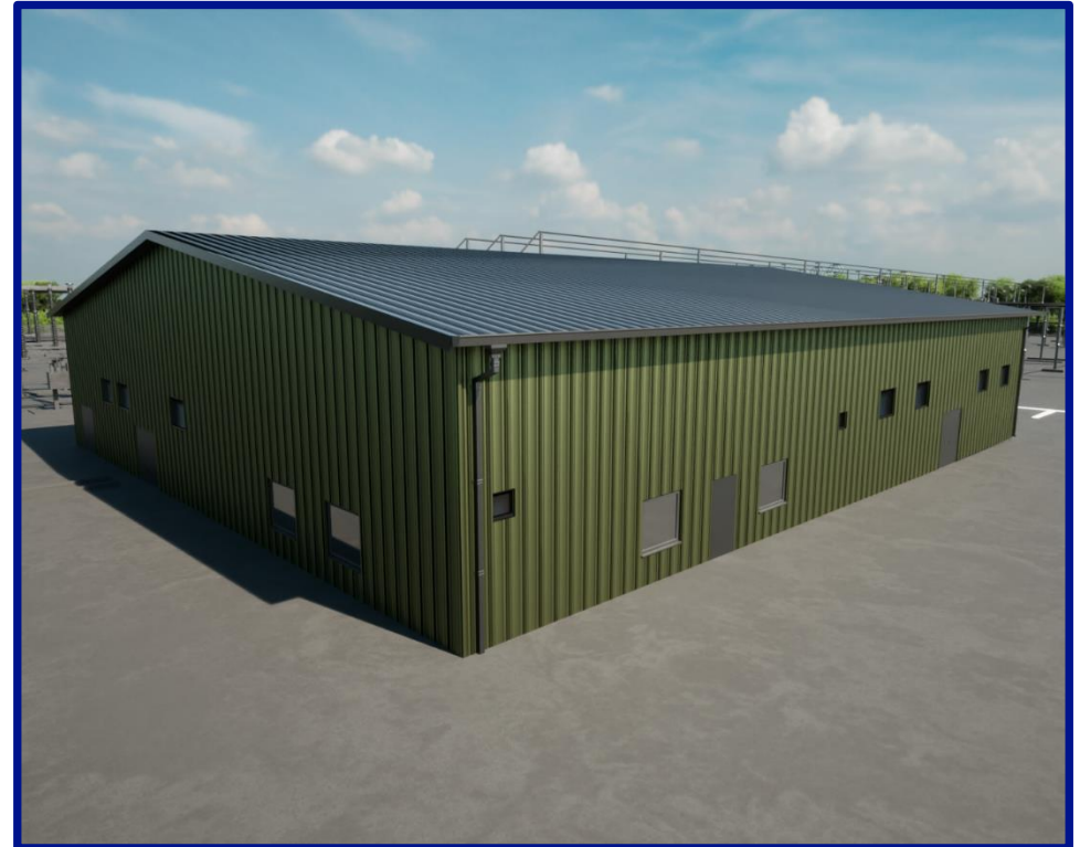
Figure 38: Monk Fyston Control Building Finish - Green Cladding
