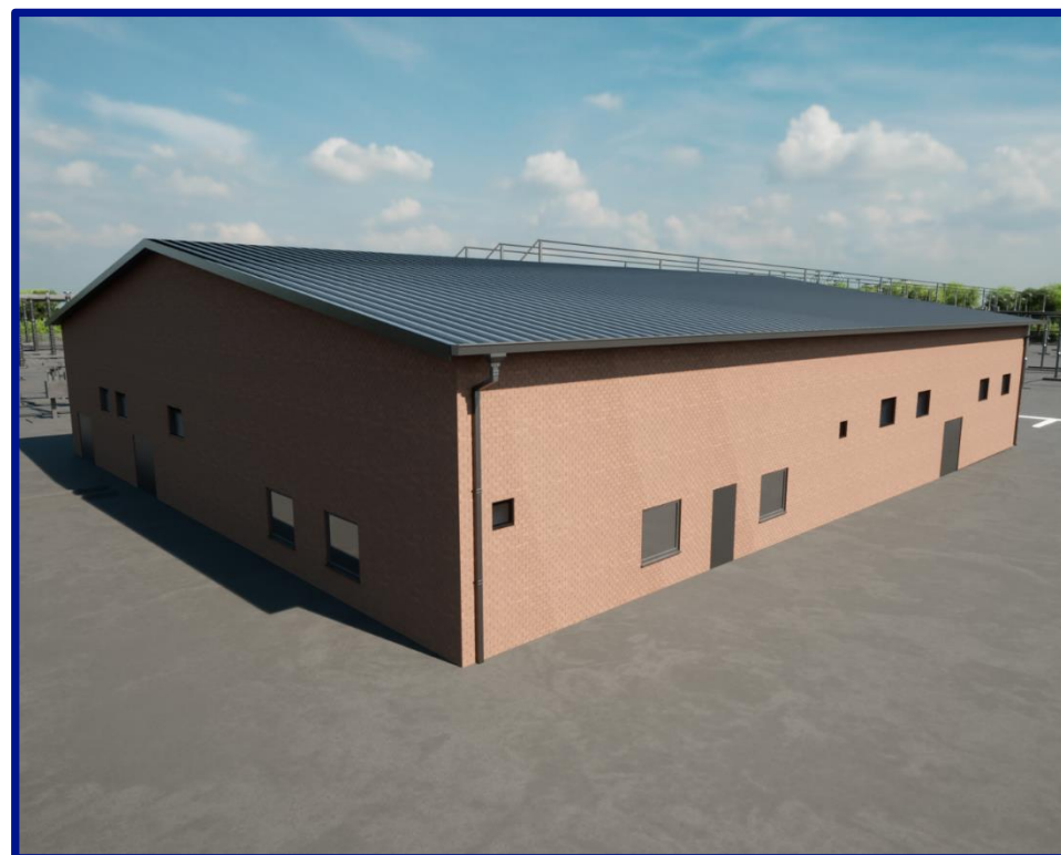
Figure 36: Monk Fryston Control Building Finish - Red Brick
