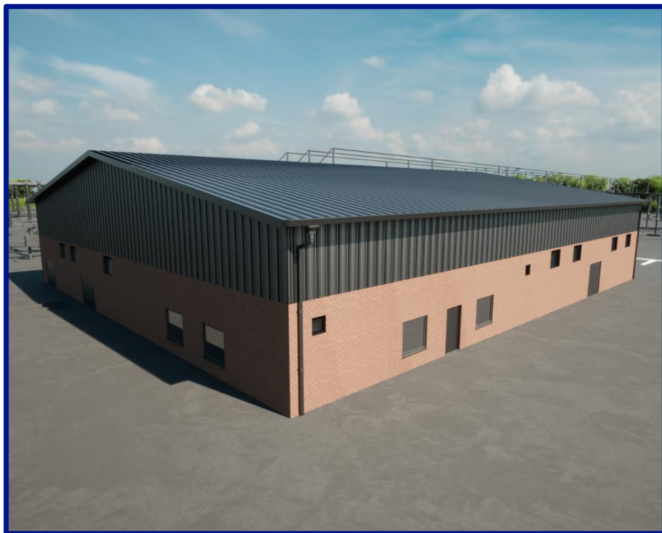
Figure 35: Monk Fryston Control Building Finish - Cladding and Red Brick
